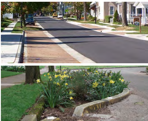
Fig. 21 Examples of curb bumpouts from Dublin, OH and Philadelphia, PA designed to calm car traffic and absorb stormwater runoff.
