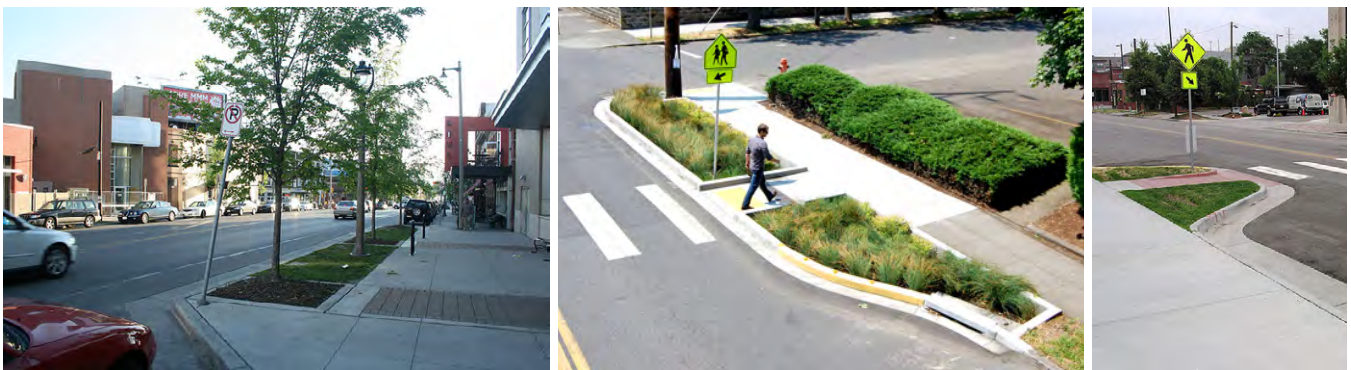
Fig. 61 Examples of vegetated curb bumpouts
