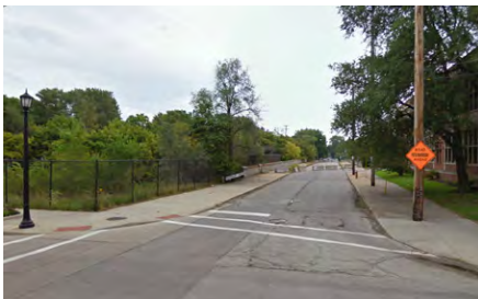
Fig. 71 Current entry to RTA Station on Madison Ave. is hidden from W. 65th St.
