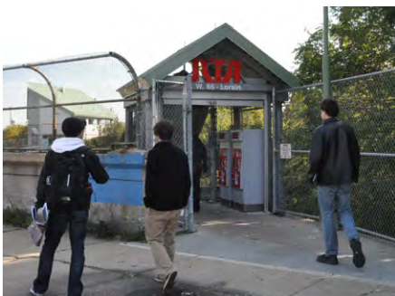
Fig. 72 Entry stairway to RTA platform
