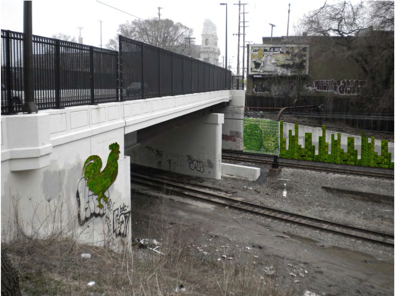
Fig. 33 Proposal showing green moss graffiti applied to the walls along the rapid corridor beneath the W. 65th St. bridge
